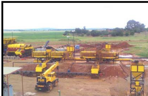
Installation of four sixteen foot pan plants
